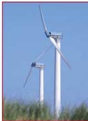
Lagerwey bipale 250kW
