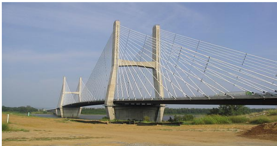
Figure I.19 : Pont Bill Emerson Memorial, Missouri, USA
