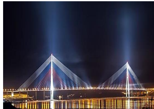
Figure II.1 : Pont de Sutong, Chine
