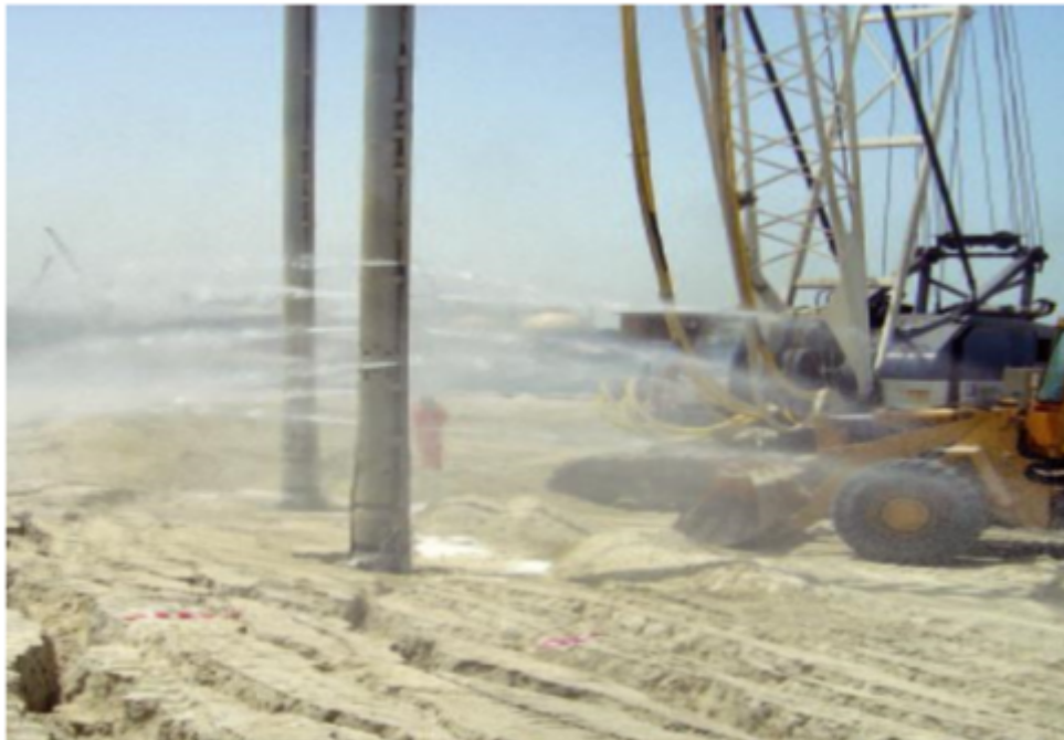
FIGURE 3.7: La vibroflotation.[7]
