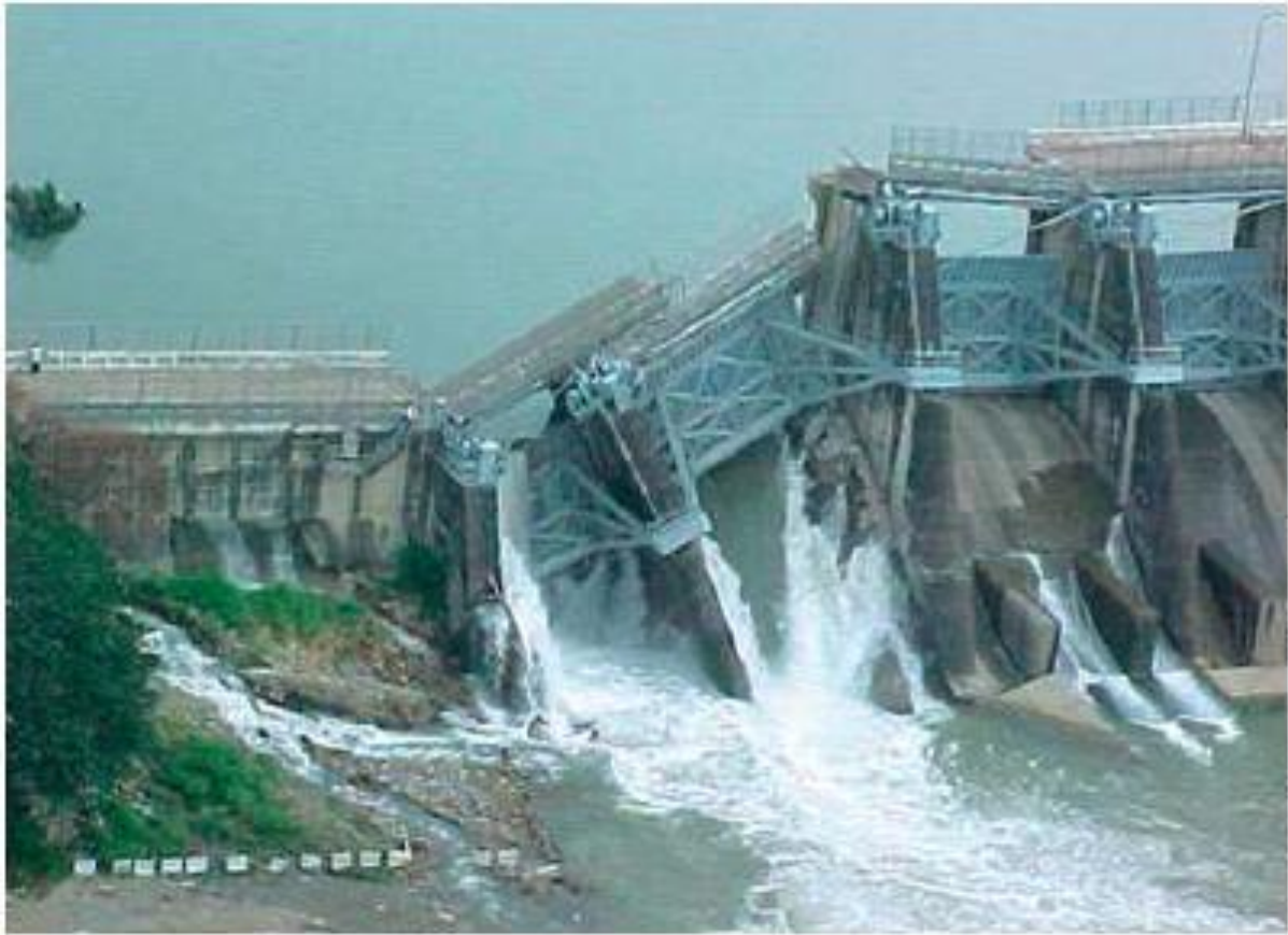
Figure I-10: Rupture du barrage de Shih-Kang (Taiwan 1999)
