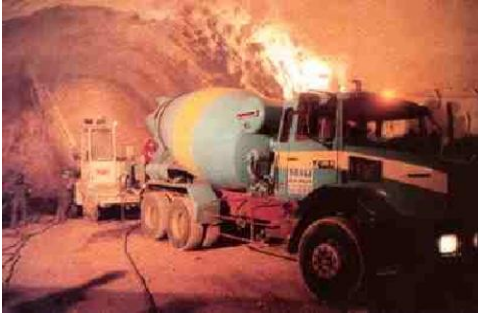
Figure II.11 :Projection du béton[WEB09]
