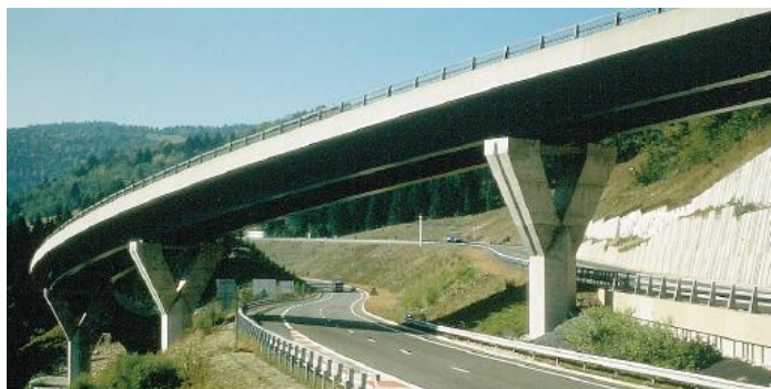
Figure. I.22. Pont bipoutre courbe [3]
