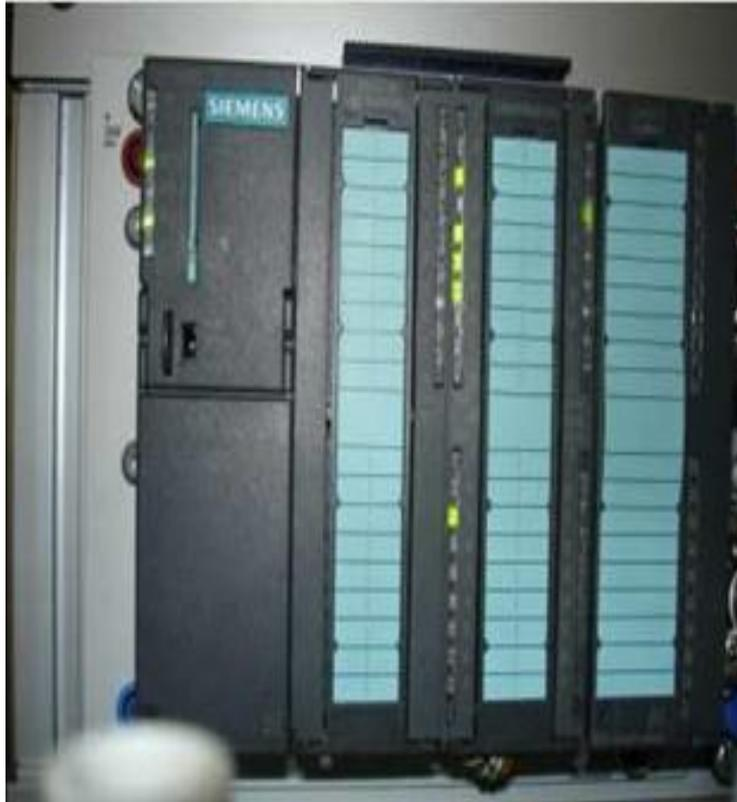
**Figure I-6 Automate S7 313C**
