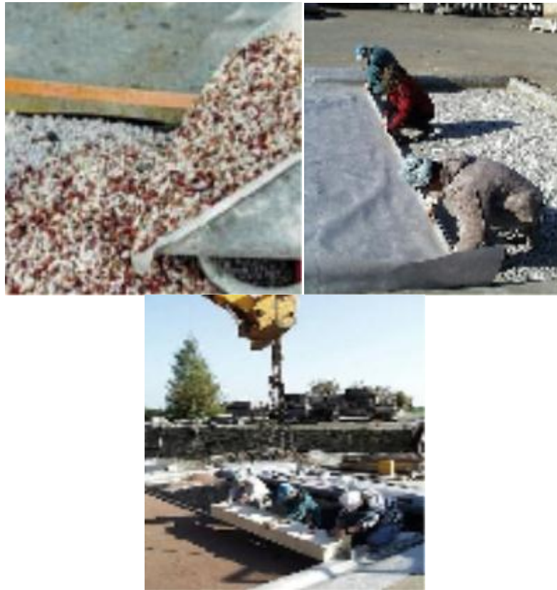
Figure III-8 Application du béton drainant.
