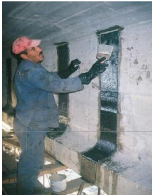
Figure III.3: Application de la couche de fermeture.
