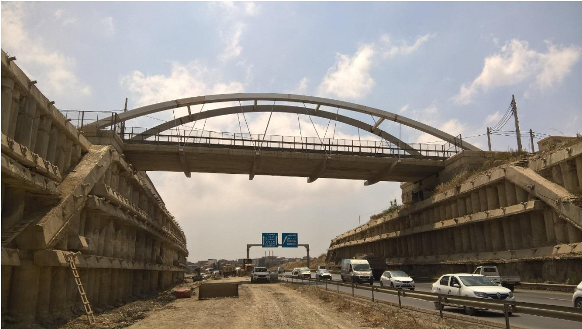
Figure IV.7: Pont de OULED MOUSSA.
