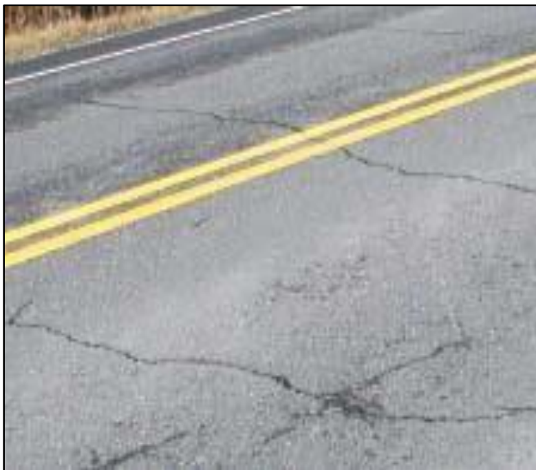
Figure1.9. Fissure transversale [54]
