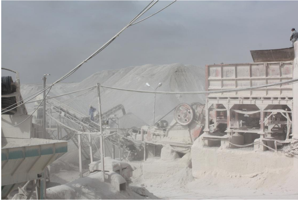
Figure II.8 : Station de concassage
