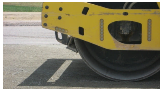
Introduction de micro-fissure
