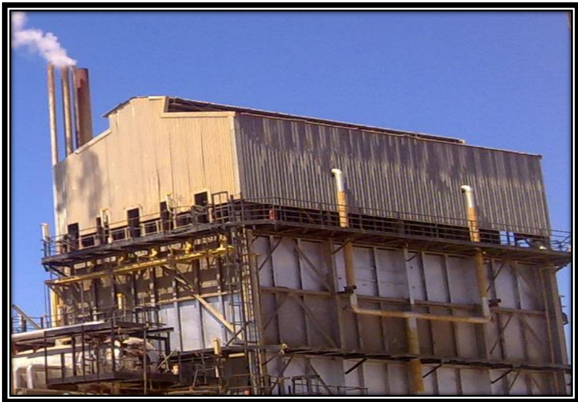
Figure VI. 3 : Four de steam reforming.
