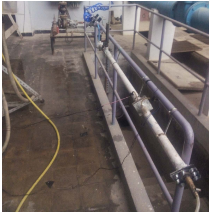
Figure 2.8: The differential pressure flowmeter with pressure transducer.
