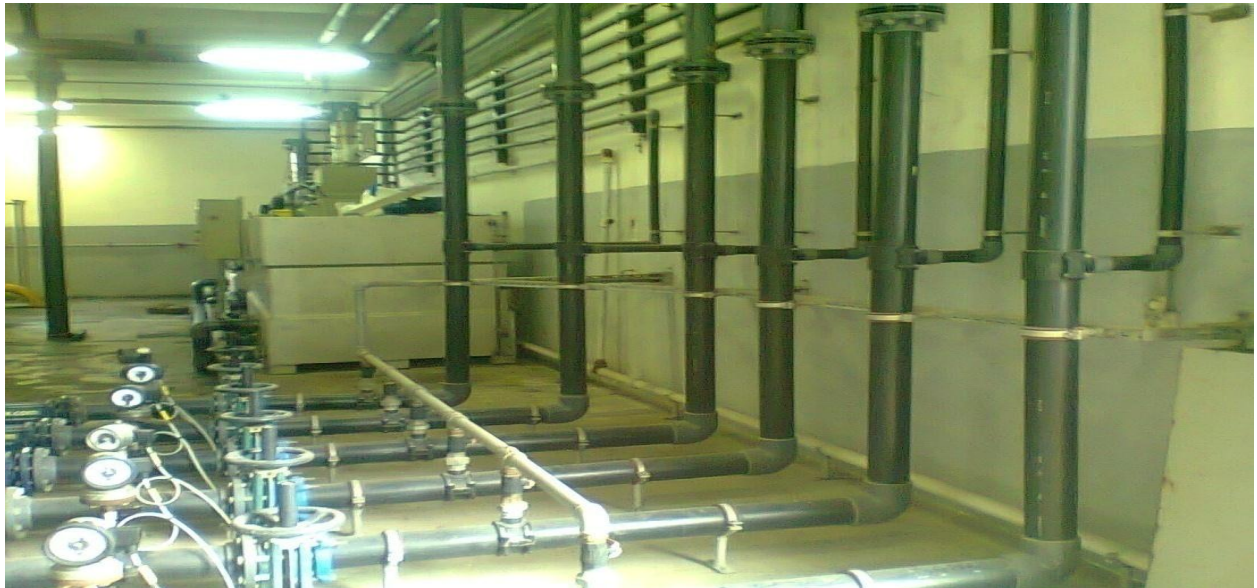
Figure II.15: Injection des polymères
