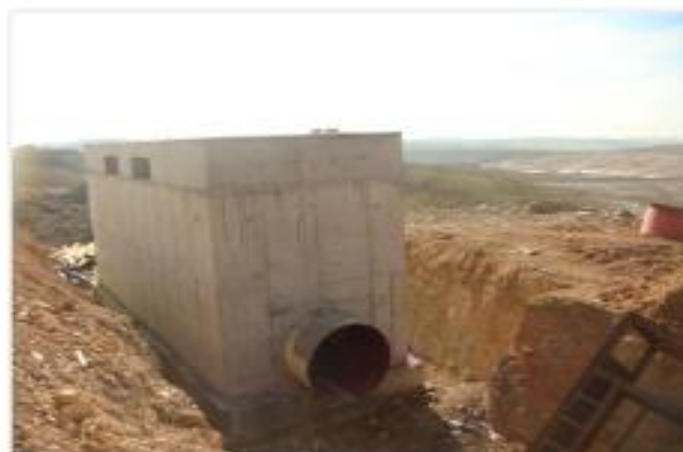
Figure VII. 5: construction des regards
