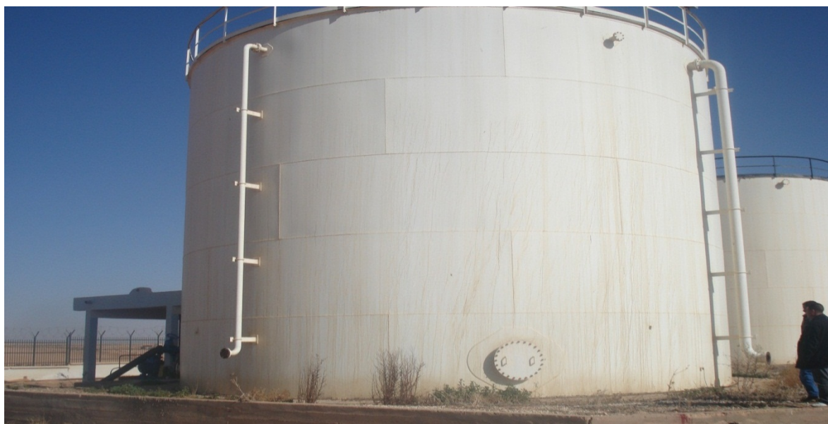
Figure III. 2 : la station de pompage sud SP122
