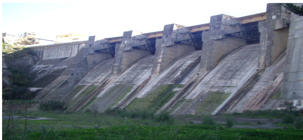
Figure III.3 : barrage de K'sob
