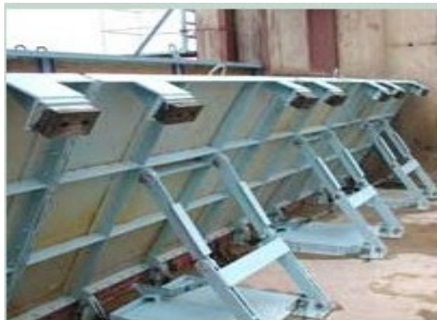
Figure III.14 : hausse rabattable
