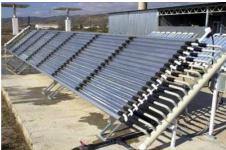
Figure 11: Modèle de Compound parabolic collector.
