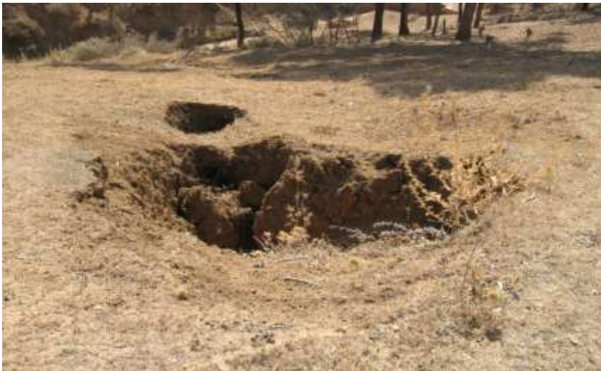
Figure I.6: Erosion en tunnel (suffosion) sur formation
