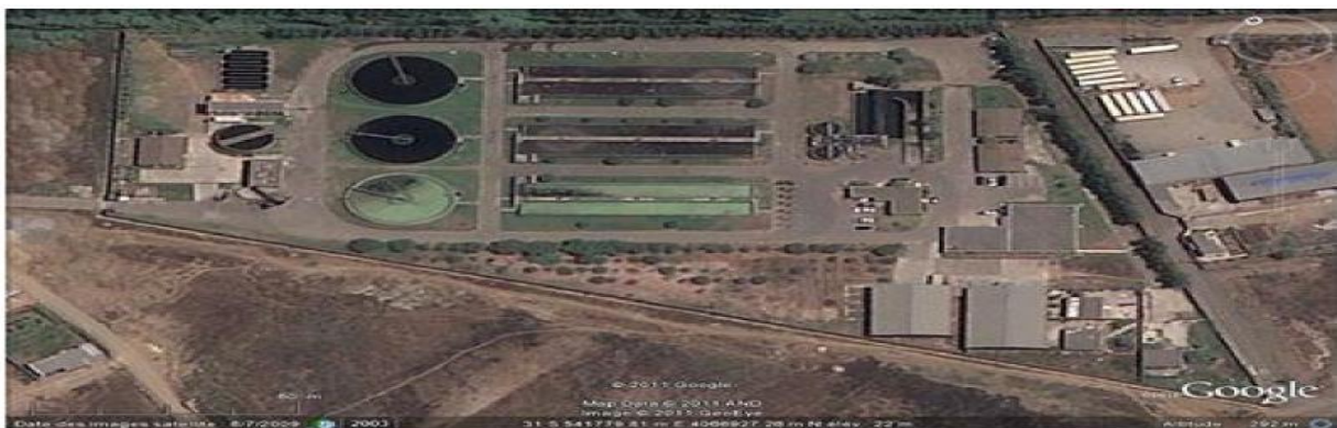
Figure III.2: STEP de Boumerdes [Google Earth]
